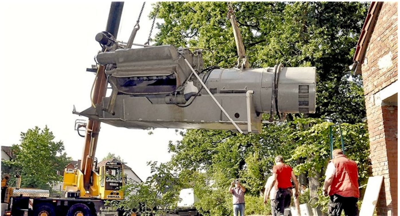
Abb. 4: Notstromaggregat
